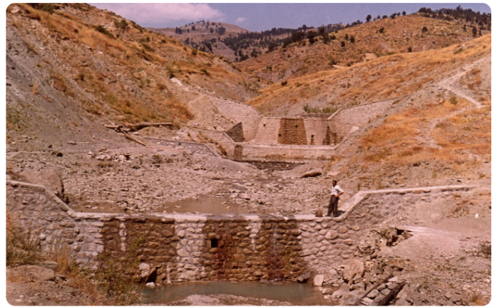
A 1960 photo showing a series of water flow control dams. A proudly standing forest guard on the dam shows the scale.
